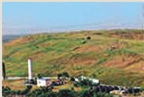
Closer & extraction of methane gas at gorai
