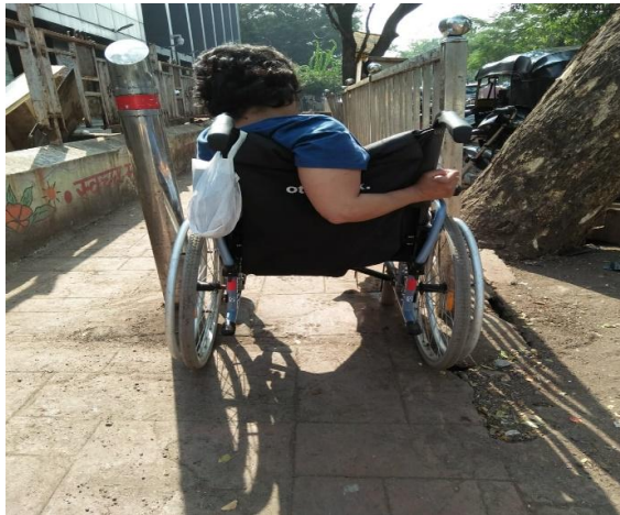
Incorrect placement of bollard create Wheelchair access impossible.
