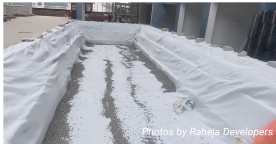
Image 3C: Geotextile fixing over the drain cell
