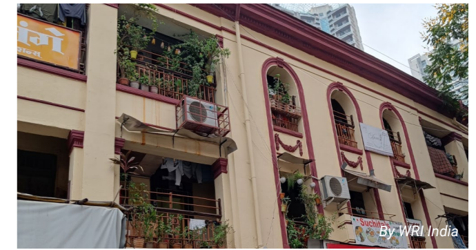
Image 2C: Container planting on projected floor slab
