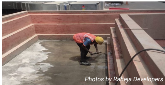
Image 3A: Waterproofing for green roof
