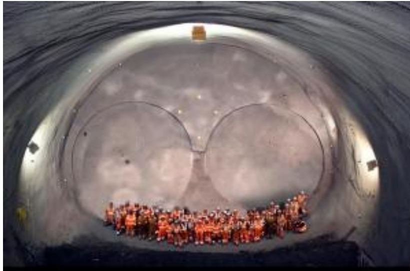
Figure 5-3 Twin TBM Bores Opening into Cavern
