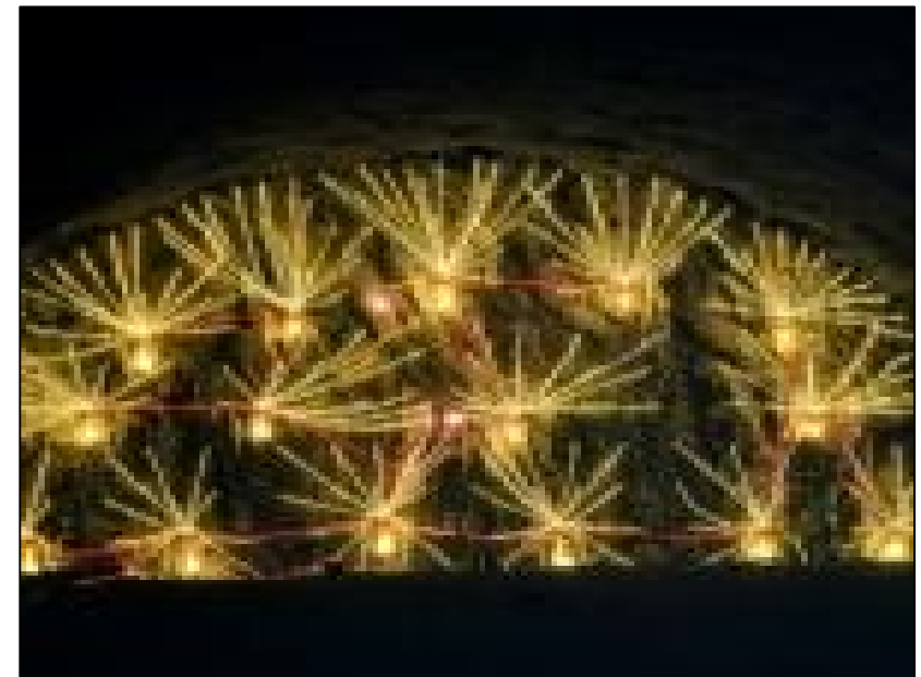
Figure 5-4 Lighting Up the Face as D&B Tunnel Shot-Fires
