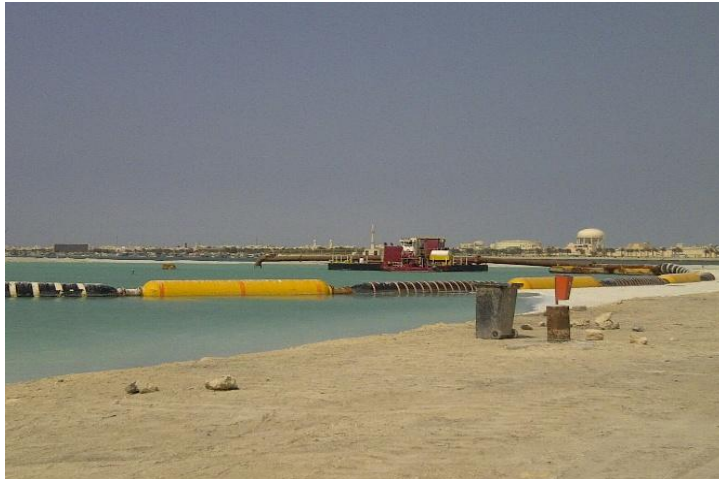
Figure 4-19 Pump Line for Hydraulic Fill Bahrain
