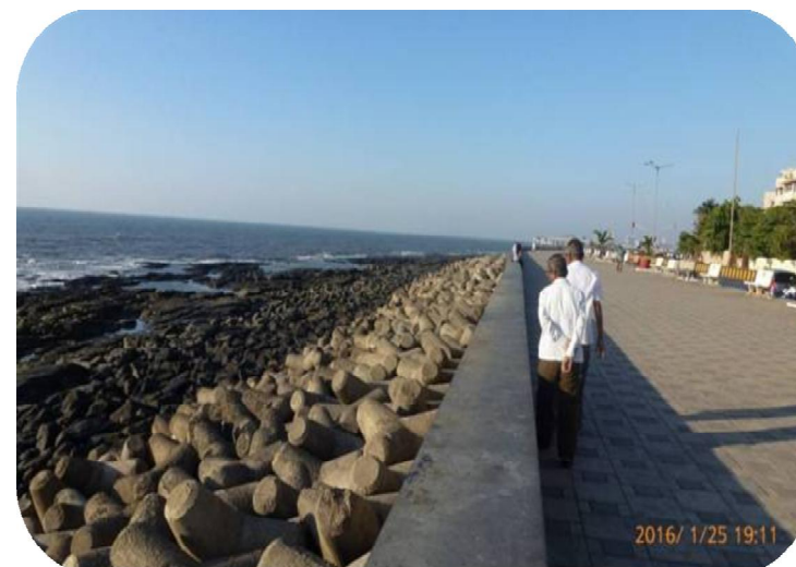
Figure 4-4 Tetrapod Protection with Concrete Capping Wall
