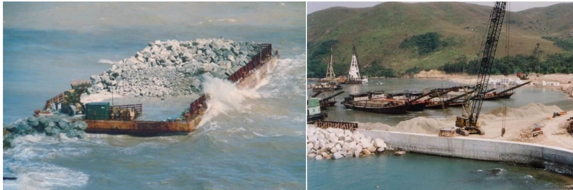
Figure 4-10 Delivery of Rock Products from Sweden to the UK & Motorised Barges Delivery of Reclamation Fill in Hong Kong
