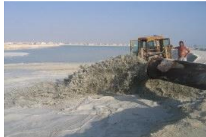
Figure 4-20 Hydraulic Filling Bahrain
