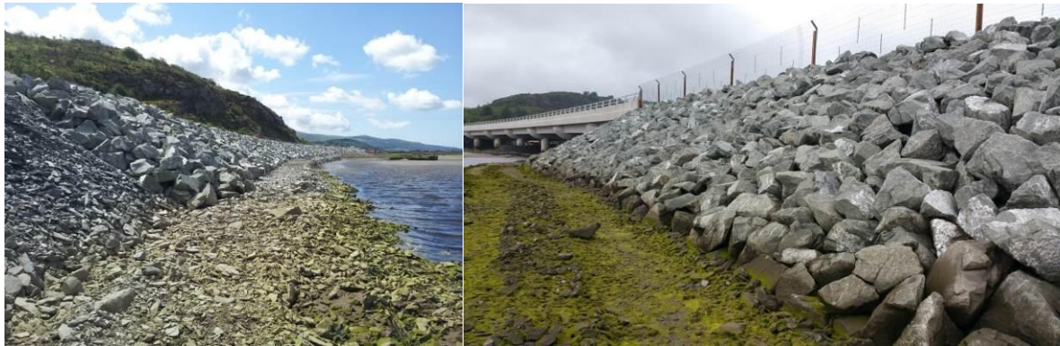
Figure 4-8 One Tonne Rock Armour Revetment & Rock Core at Low Tide Pont Briwet Wales (Locally Delivered Basalt)
