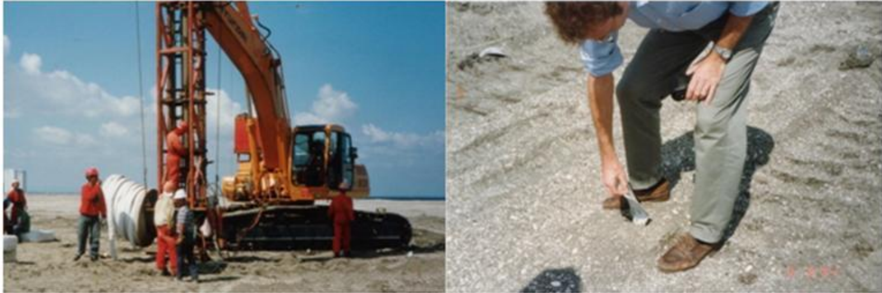
Figure 4-15 Installation of Wick Drains (Central Area Reclamation Manila)
