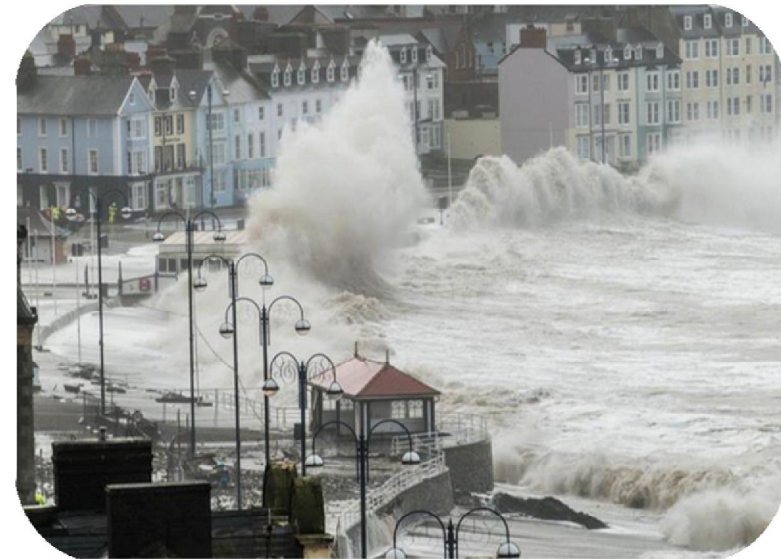
Figure 4-6 Wave Overtopping
