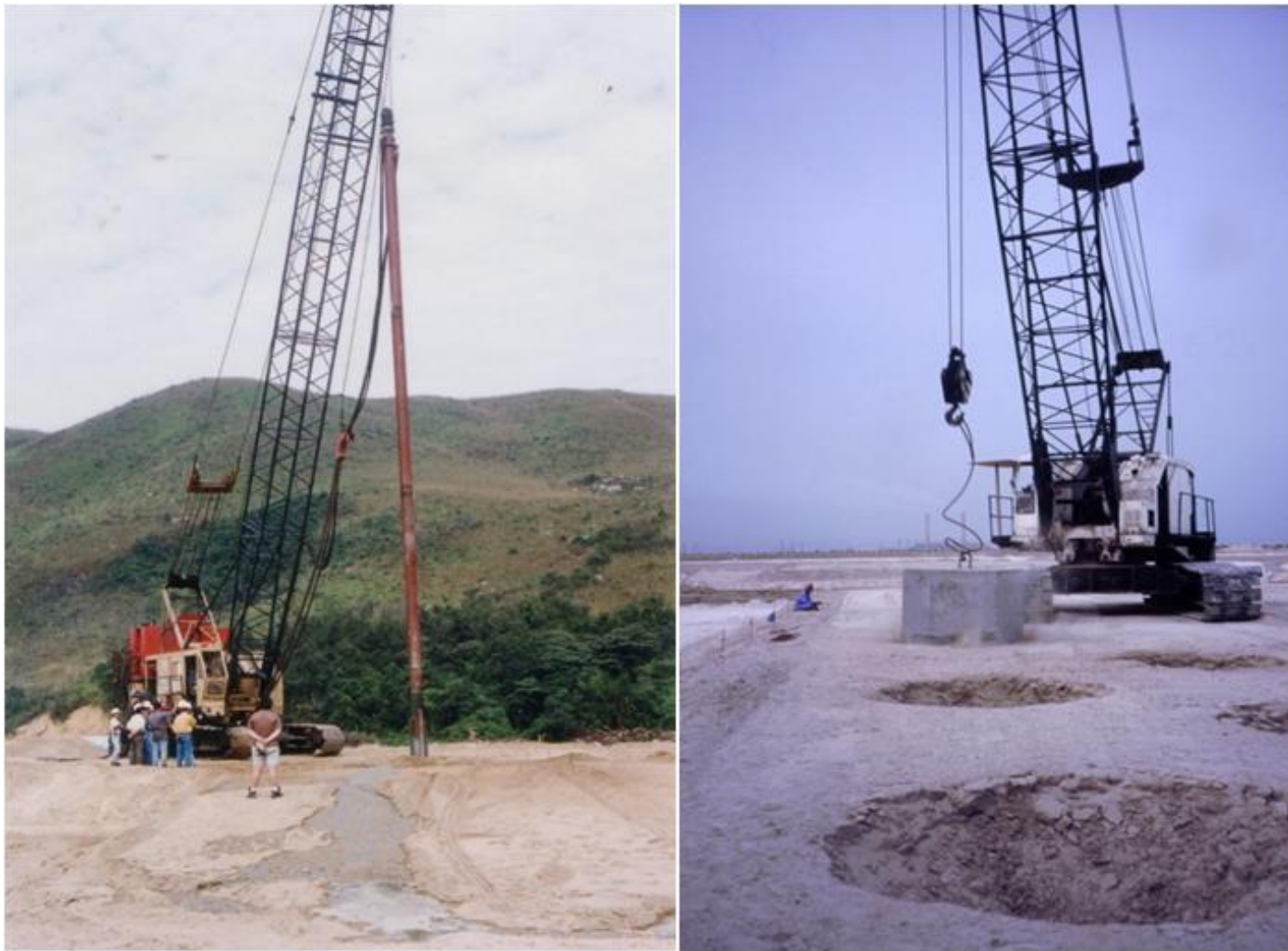
Figure 4-16 Vibro-Compaction Lantau Island Hong Kong & Dynamic Compaction at Al Khiran in Kuwait Materials Specifications
