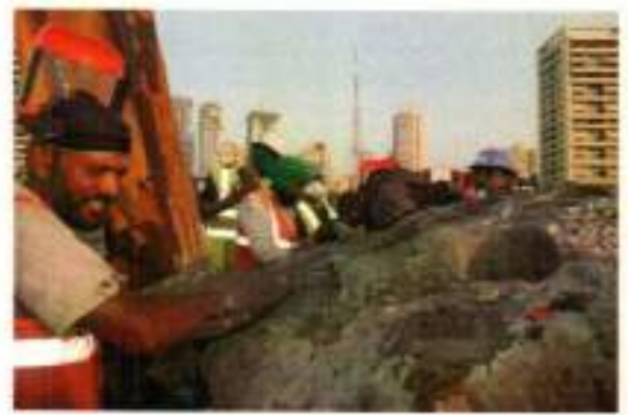
Picture_ 5 Placement of Coral on Rock (Fixing)
